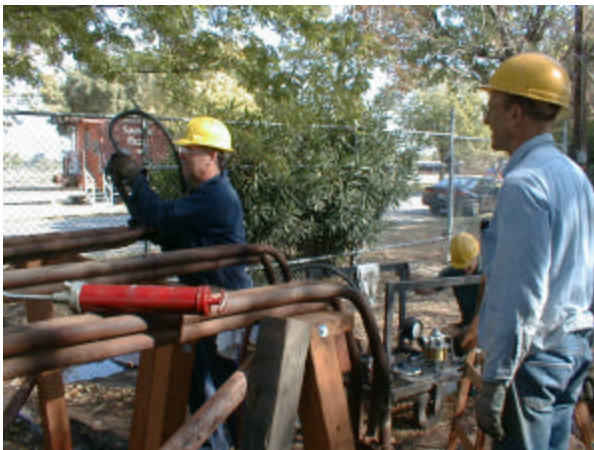
Testing the superheater tubes with pressure
