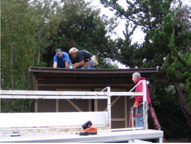
Re-papering the Outfitters shack roof
