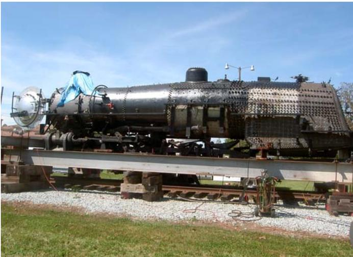
finish in the next month: 3 flexible stay bolt half sleeves, 1 Full sleeve and the installation of a flexible stay bolt, 2 Ridge staybolts in the side sheet and the installation of a bushing on the back head for the water column with these repairs the boiler will be a pressure vessel again.
