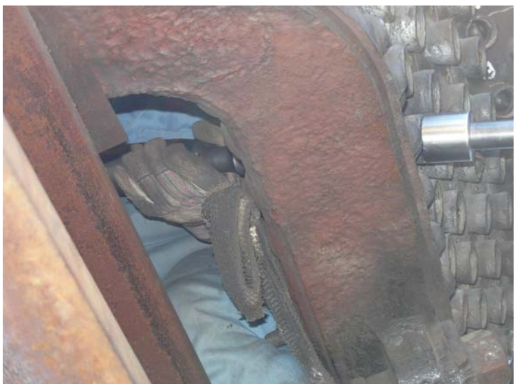
Showing the bucking hammer on the left and the bar tool on the right
