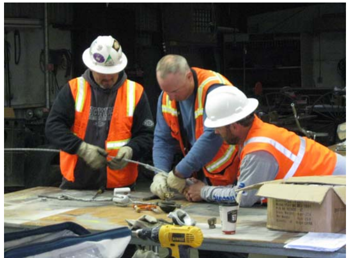
Pre Assembly of cross arm hardware
