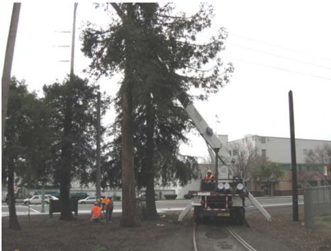
Installing first Steel Pole
