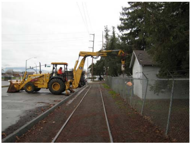
Drilling a hole in tight places
