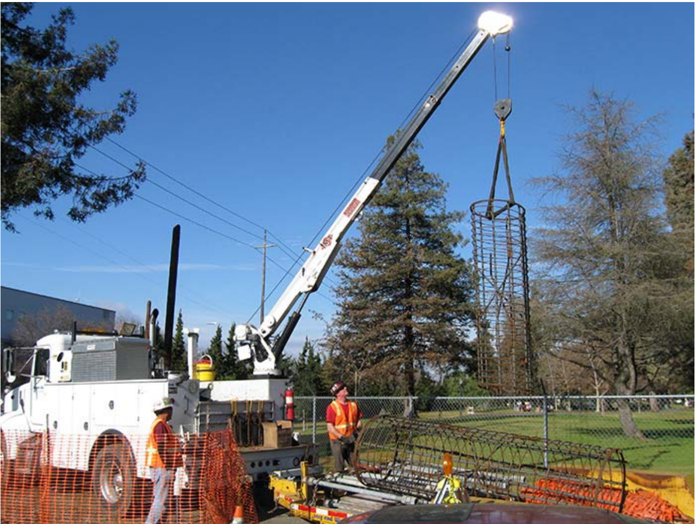
Inserting reinforcing steel in three foot diameter hole
