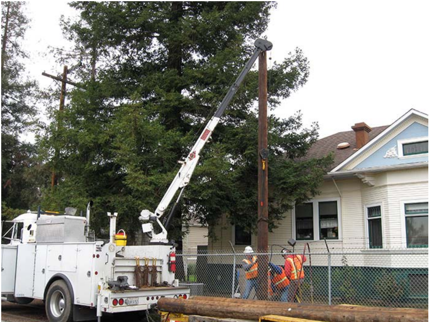
Installing a Pole
