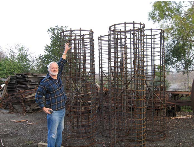
Steel Reinforcing for iron pole foundation
