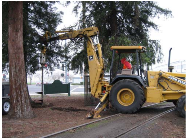
drilling three foot diameter hole for steel poles
