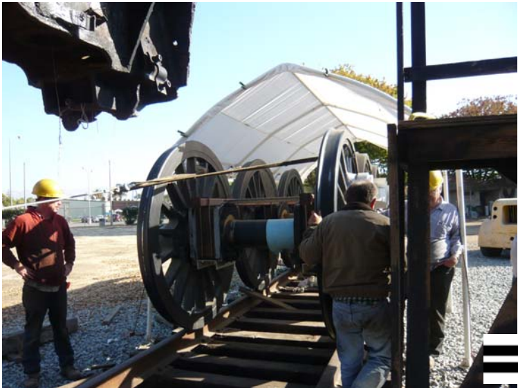
Pulling the wheels toward the locomotive
