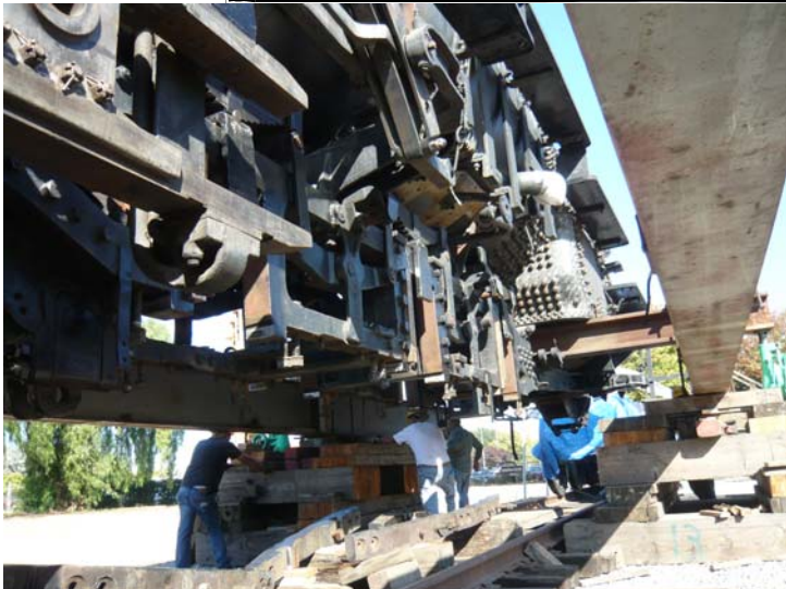
Working under the locomotive
