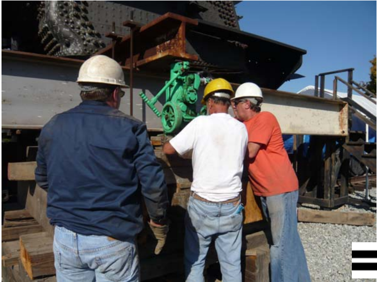
Preparing to lift the locomotive
