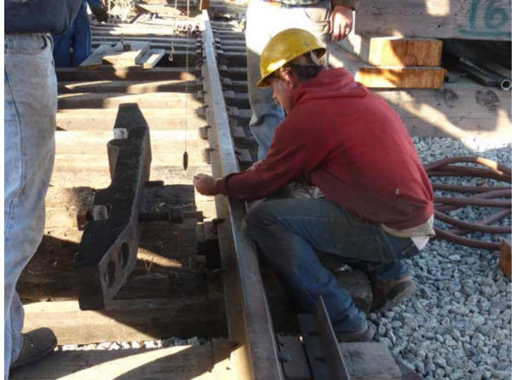
Aligning the frame with the rails
